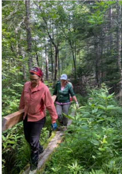
All trail work photos by Phil Coyne
